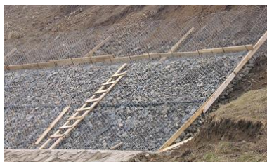
http://lt.lt.allconstructions.com/portal/categories/309/1/0/1/article/18712/gabionai-kas-tai-yra-ir-kur-naudingi pav. Pintos vielos tinklas šlaito sutvirtinimui
